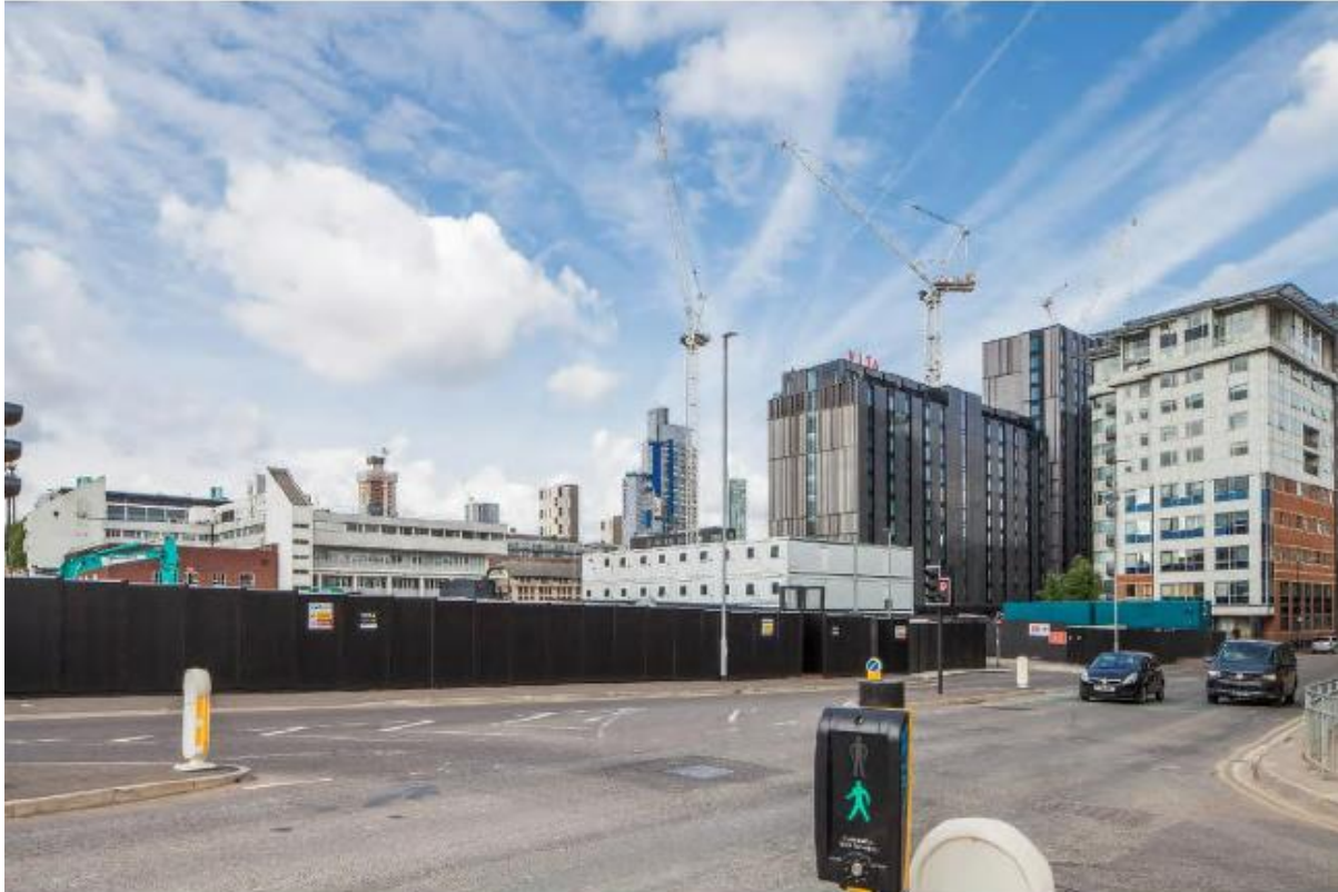
Viewpoint 11 – Brook Street (existing)
